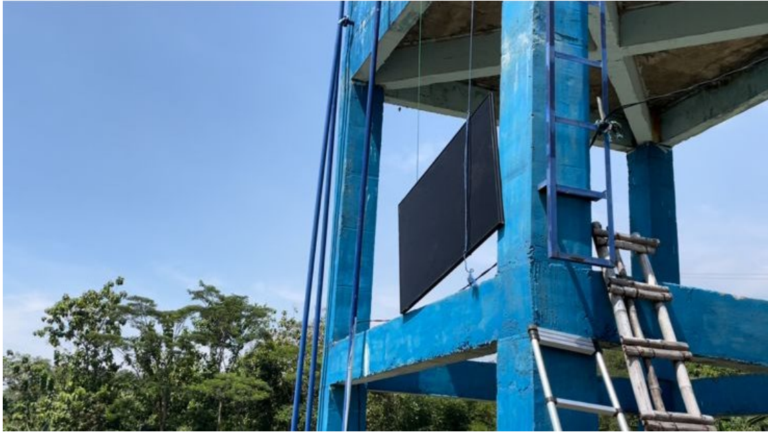
Figure 8. The process of installing solar panels onto the substation
