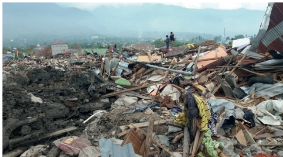
Figure 1. Ruined houses at Balaroa, as impacted by liquefaction following Palu earthquake
