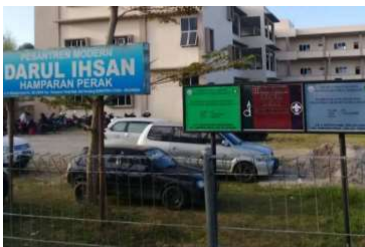
Figure 1. Darul Ihsan Islamic Boarding School, Deli Serdang
